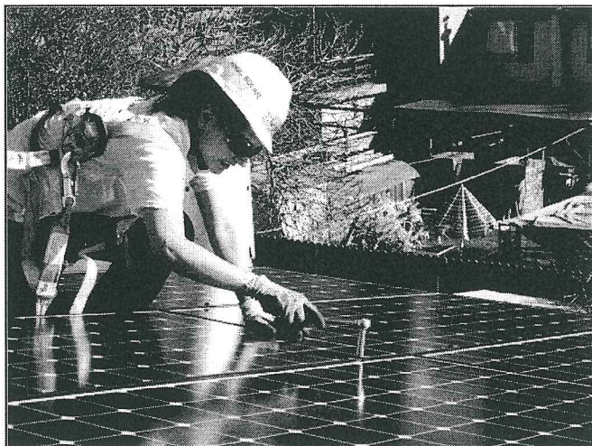
ERG solar panel installation in Richmond, CA
